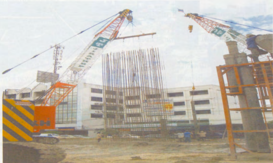
Supports for Reinforcing cage
