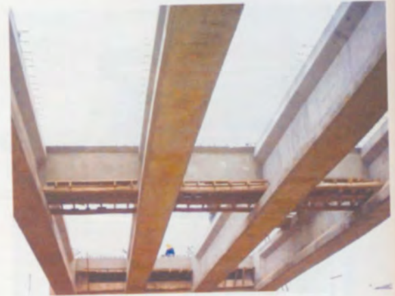
Intermediate Diaphragm
